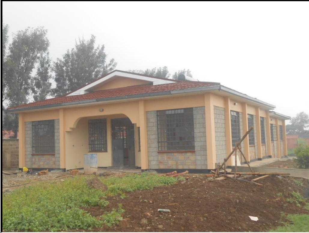
The ongoing Kitchen and Dining Project at ASN Upendo Village
